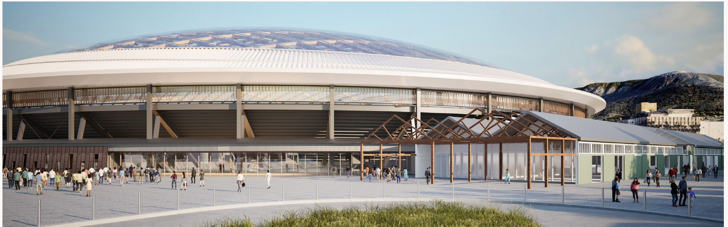
Figure 1-1: View toward the relocated Goods Shed from the northern access road.
