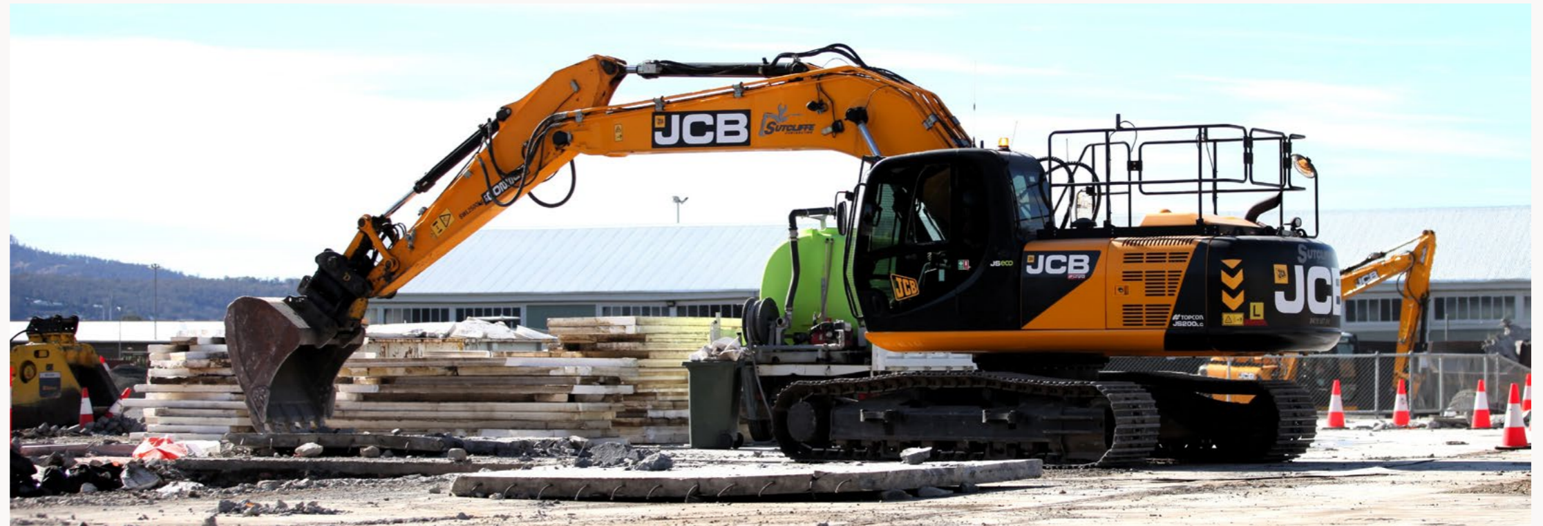
Figure 8-11: Excavator in use on Macquarie Point (Photo: K Murray-Cox 2024).
