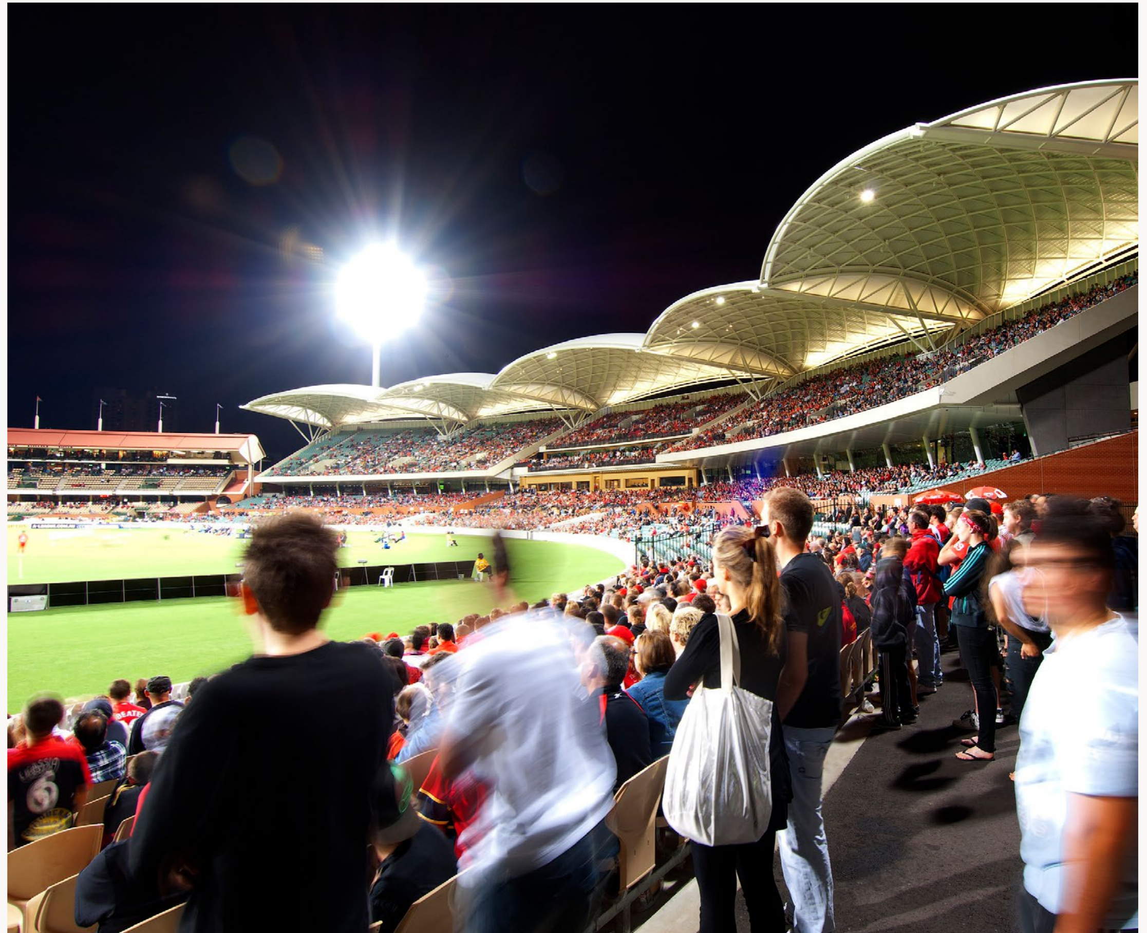
Figure 7-3: Western grandstand, Adelaide Oval.
